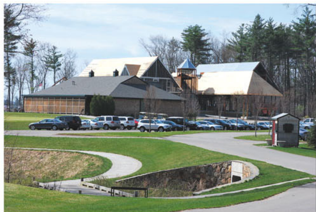
Scheduled to be completed this fall, the 30,000-square-foot clubhouse at Renaissance GC has put to rest any lingering doubts about the future of the high-end private club in Haverhill. Photo by Kevin Keller
